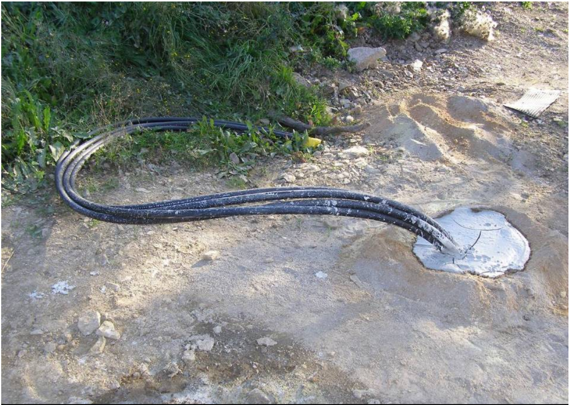
A GROUTED WELL
